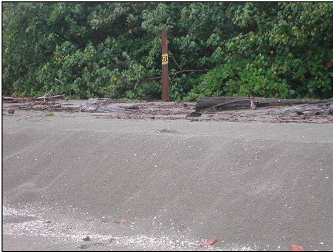
Figure 35: Beach erosion at mojon 51
