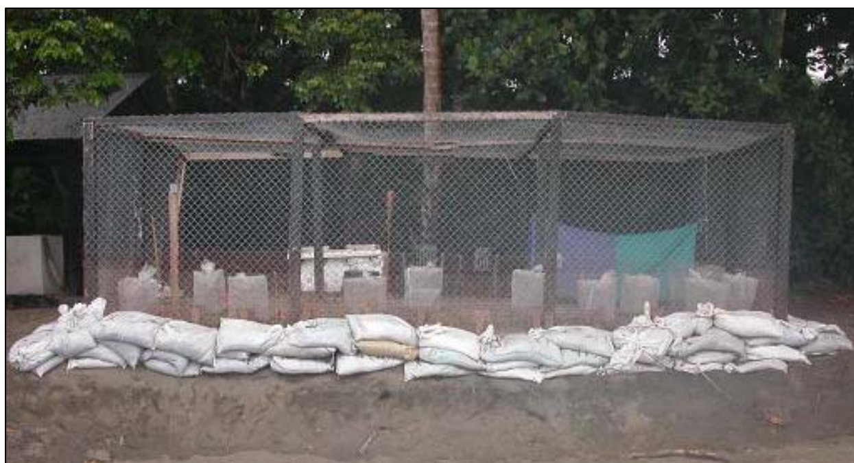
Figure 8: Front view showing moat pit and sandbags to try and prevent encroaching tides throughout the season
