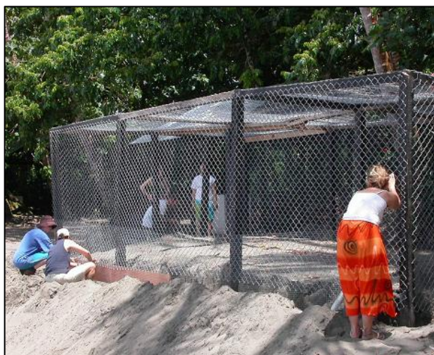
Figure 6: Volunteers assisting with the construction
